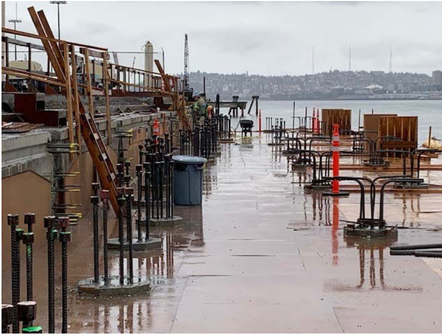
Cages in existing piles + Dowels in new piles
