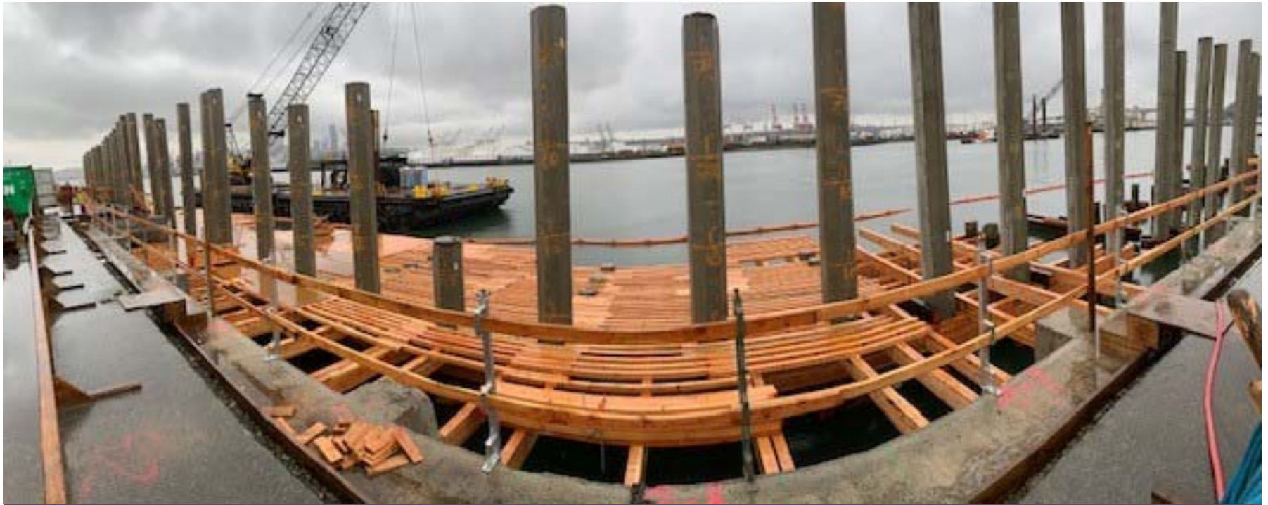
Overwater Construction: Falsework Installation of Collars, Glulam, 4X4s, Decking Fisheye view
